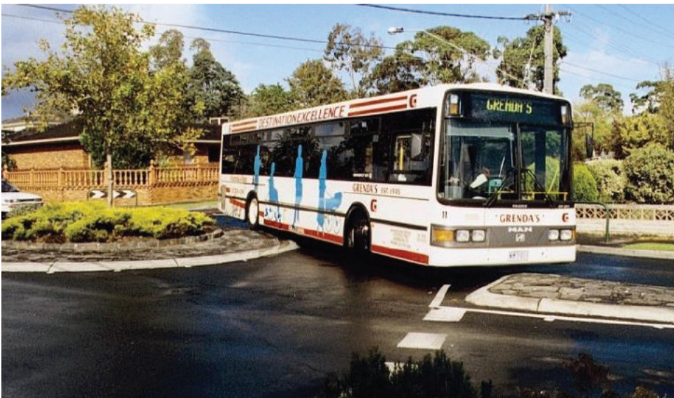
Figure 5.4.6.3: Areas behind kerbs should be kept clear of objects. Source: Austroads Guide to Road Design Part 4B Roundabouts
