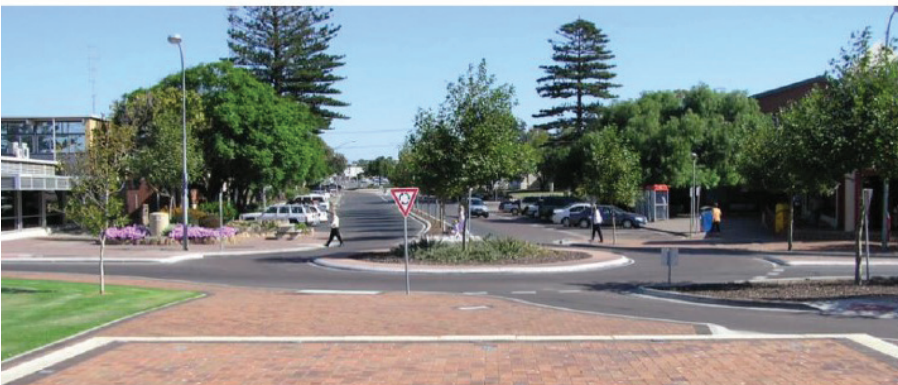
Figure 5.4.6.6: Example of a landscape treatment at a small local street roundabout Source: Austroads Guide to Road Design Part 4B Roundabouts.
