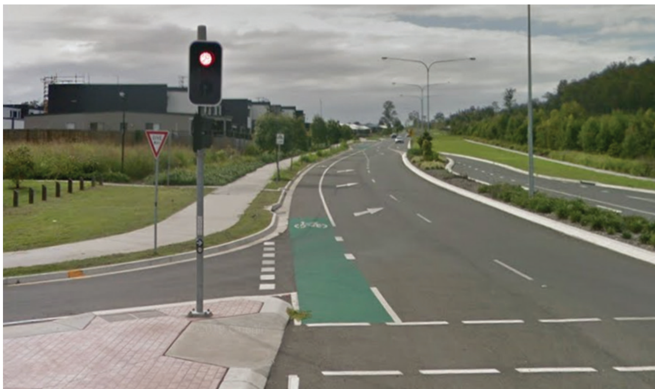
Figure 6.1.5 SEQ Regional grid watermain located under the on-road cycle-lane. (Left-turn slip lanes as shown in this Figure should be avoided - see Section 5.4.9 Signalised Crossings).
