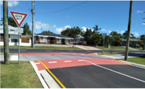
Figure 2.2.2 - Example Crossing Treatment – Raised priority Crossing
