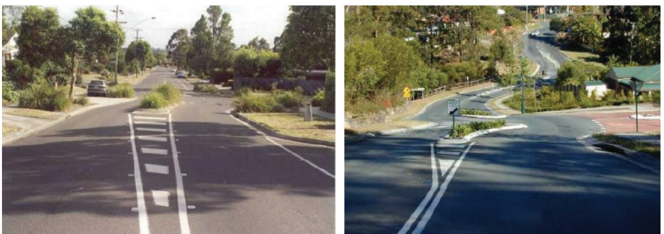
Figure 5.4.5.2: Examples of modified T-intersection channelisation. Source: Examples of modified T-intersection channelization from page 106 of Austrroads Guide to Traffic Practice Part 8: Local Street Management . Supplied by City of Monash and Moreton Bay Regional Council. .
