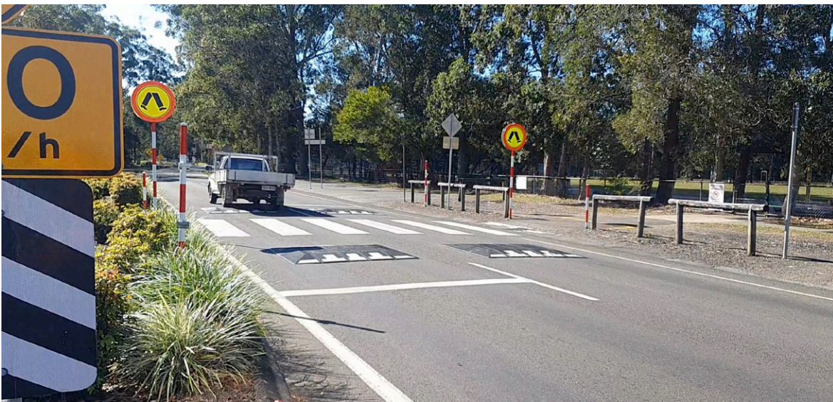
Figure 2.2.1: Zebra crossing where low vehicle approach speeds are enforced by speed cushions
