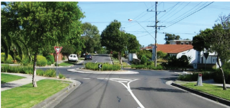
Figure 5.4.6.5: Example of a landscape treatment at a small local street roundabout Source: Austroads Guide to Road Design Part 4B Roundabouts.
