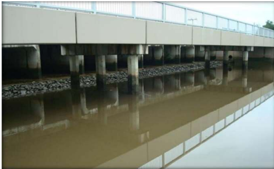
Figure 5. Upstream - Santa Barbara Culverts
