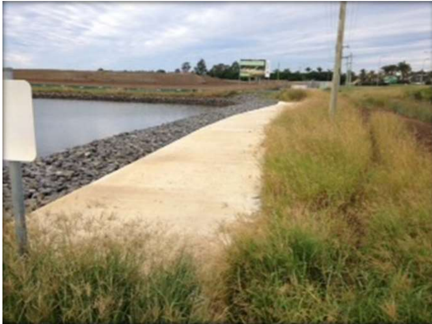
Figure 6. Downstream - Santa Barbara Culverts
