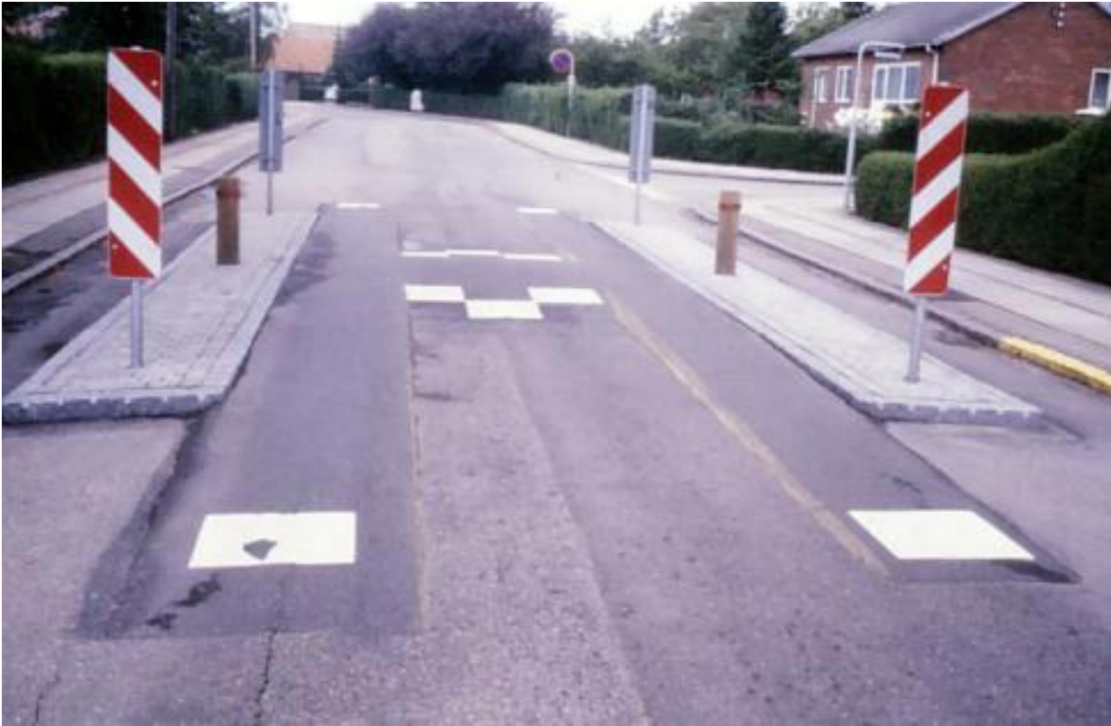
Figure 8.3: Combination road hump (Copenhagen)
